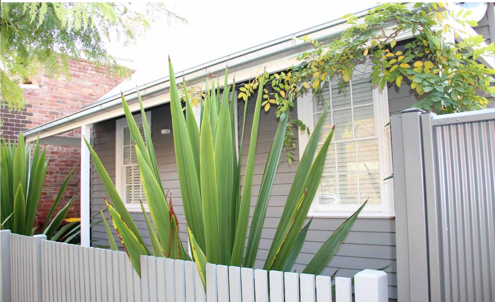
also be considered: fibre boards require vertical joints at smaller intervals than solid timber, because they may expand and contract significantly in heat and cold. Placing joints closer together reduces the risk of entire boards cracking or deforming with this movement, but breaks up the long, continuous design lines for which weatherboard is known.
